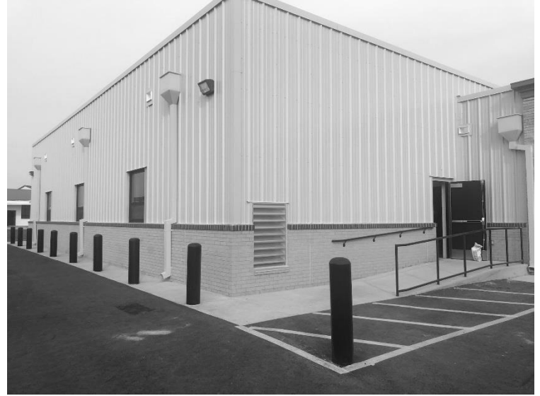
FEMA Shelter/Weight Room USD 463, attached to Middle School Gym
